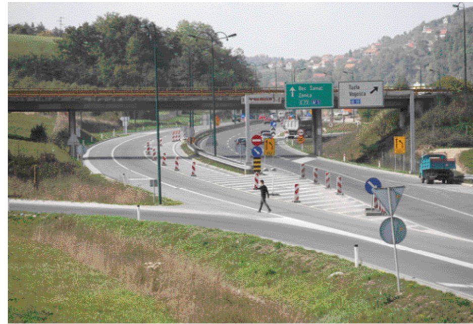
EBRD funded road project in Bosnia and Herzegovina
